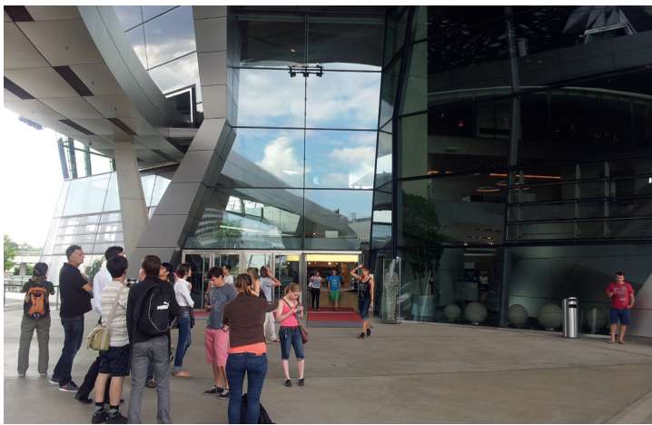
Foto: International Office
